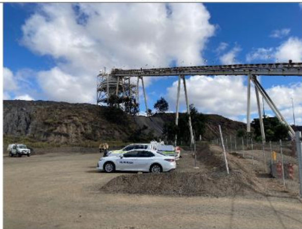
2. Conveyor belt to refuse loading area (view from CHPP carpark)
